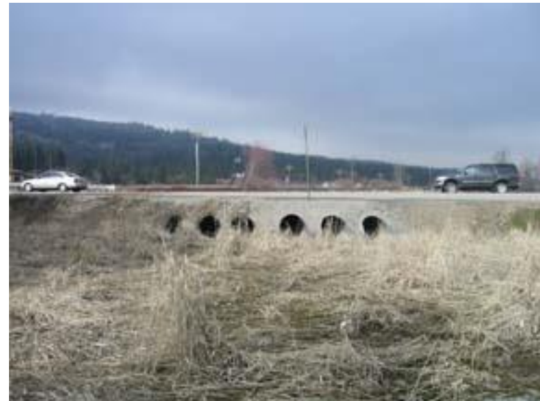
Figure 11: Dishman-Mica Road/Schafer Road. Looking at downstream face of culverts
