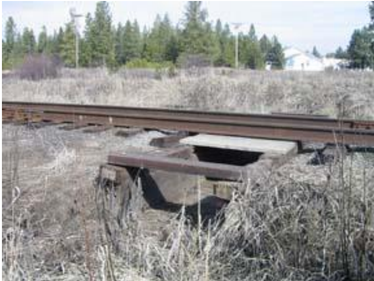
Figure 16: Culvert under railroad between Schafer and Dishman/Mica
