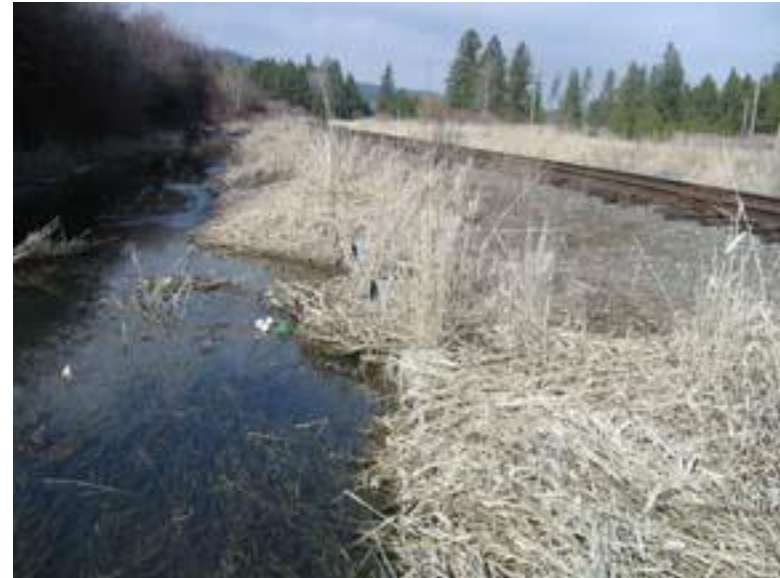
Figure 14: Culvert under railroad between Schafer and Dishman/Mica
