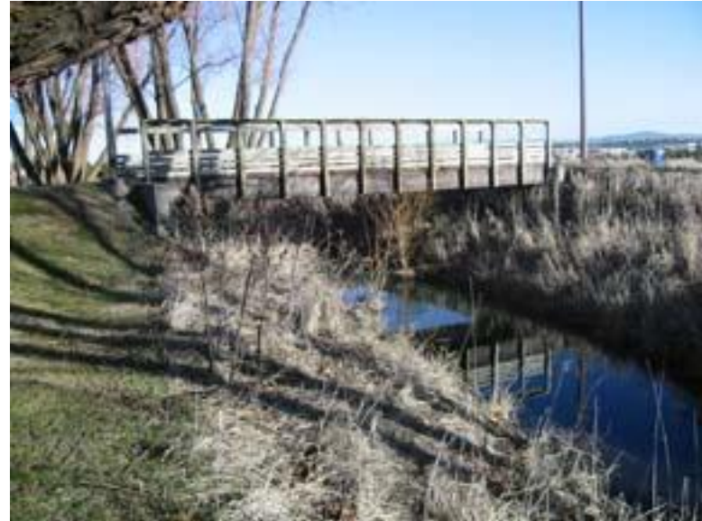
Figure 32: Footbridges on golf course. Looking at upstream face of upstream footbridge
