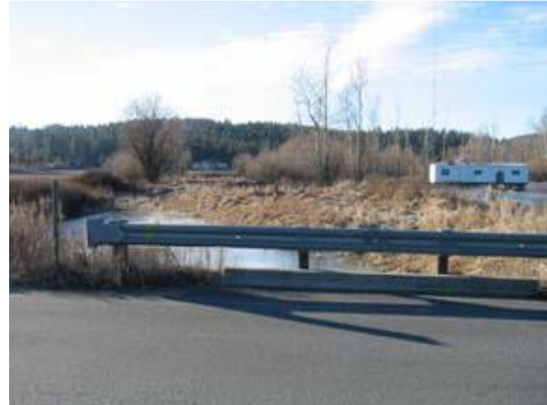
Figure 36: Thorpe road clear span. Looking upstream from bridge
