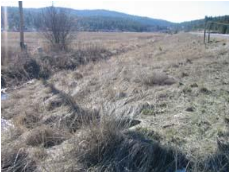
Figure 62: HWY 27 culvert. Looking upstream
