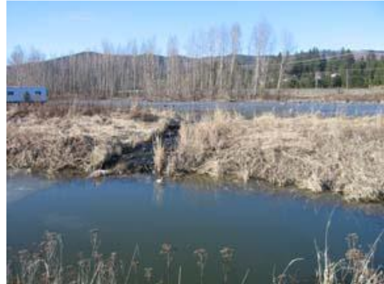
Figure 40: Spillway from pond. Drains along left bank about 50' upstream of Thorpe road
