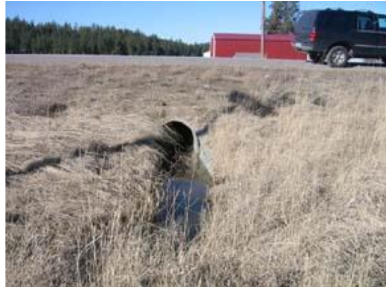
Figure 63: HWY 27 culvert. Looking at upstream face of culvert
