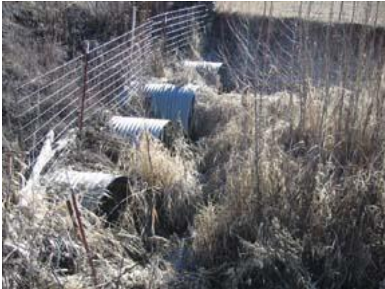
Figure 47: Chester Creek Lane. Upstream face of culverts
