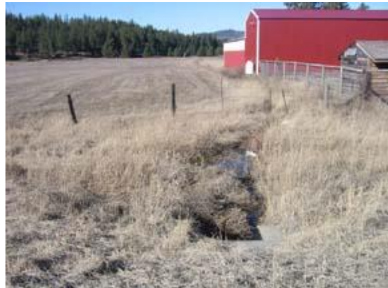
Figure 64: HWY 27 culvert. Looking along downstream channel
