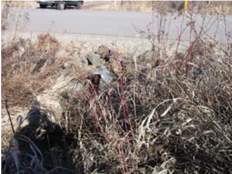
Figure 61: 46th Avenue. Looking at upstream face of culvert
