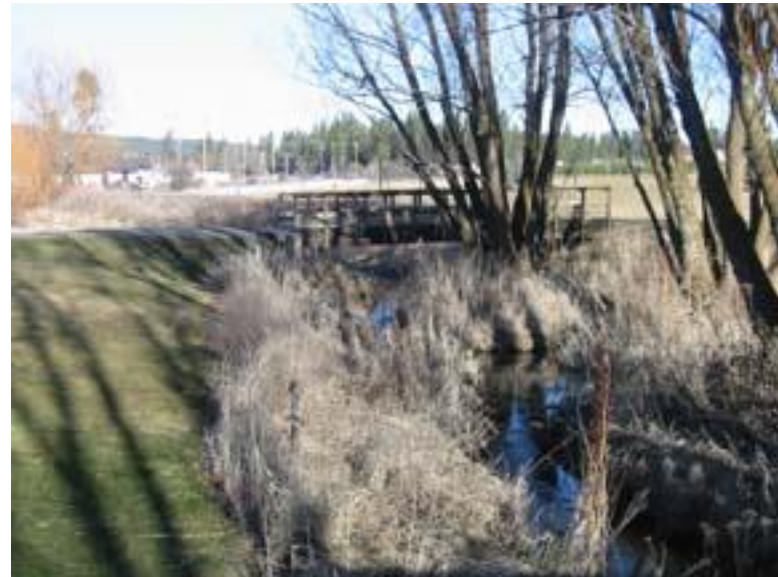
Figure 33: Footbridges on golf course. Looking at upstream face of downstream footbridge
