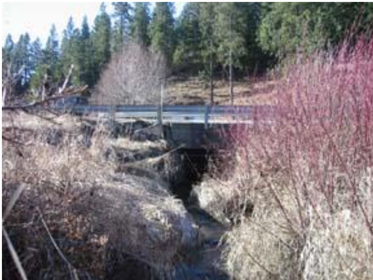
Figure 51: Dishman/Mica Road. Looking at downstream bridge face
