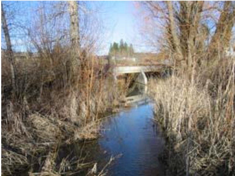
Figure 31: Dishman-Mica road crossing. Looking at upstream bridge face
