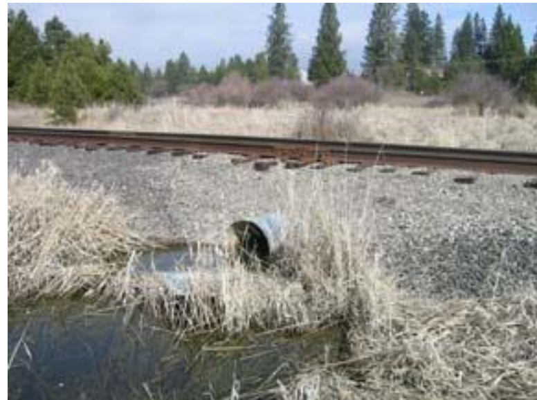
Figure 19: Culvert under railroad between Schafer and Dishman/Mica
