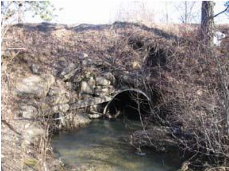
Figure 43: Mohawk road. Looking at upstream face of culvert
