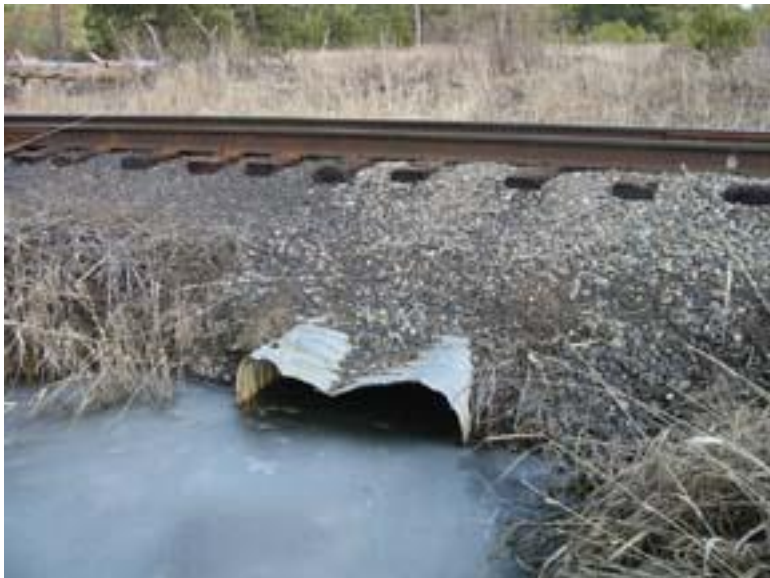
Figure 17: Culvert under railroad between Schafer and Dishman/Mica
