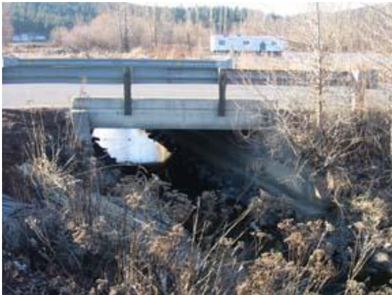
Figure 39: Thorpe road clear span. Looking at downstream bridge face
