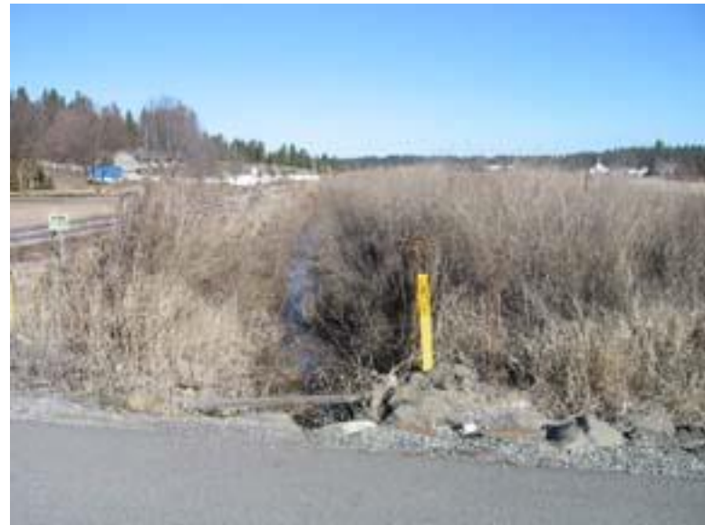
Figure 60: 46th Avenue. Looking downstream
