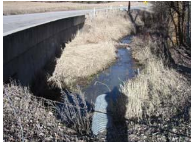
Figure 57: Dishman/Mica Road. Looking at downstream bridge face and downstream channel
