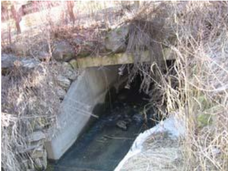
Figure 54: Dishman/Mica Road. Looking at downstream bridge face
