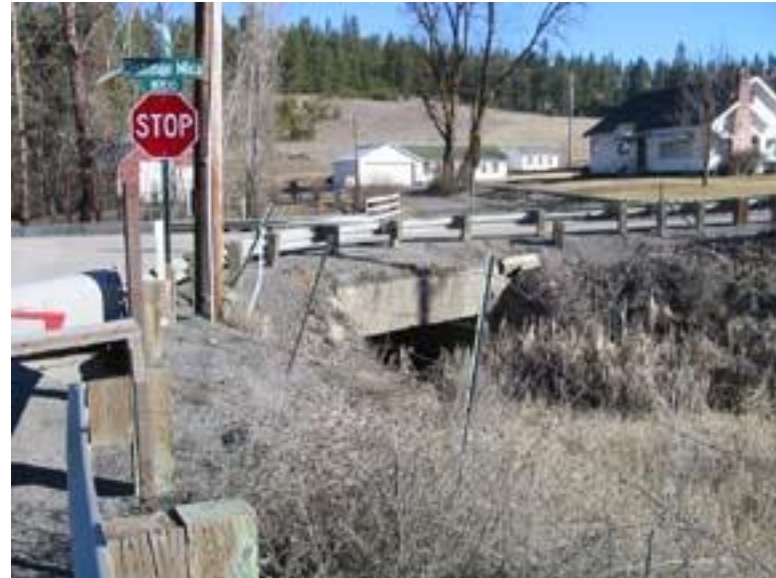
Figure 56: Dishman/Mica Road. Looking at upstream bridge face
