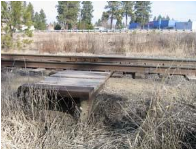
Figure 13: Culvert under railroad between Schafer and Dishman/Mica
