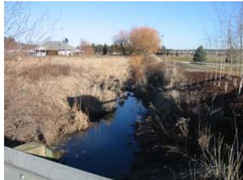
Figure 37: Thorpe road clear span. Looking downstream from bridge
