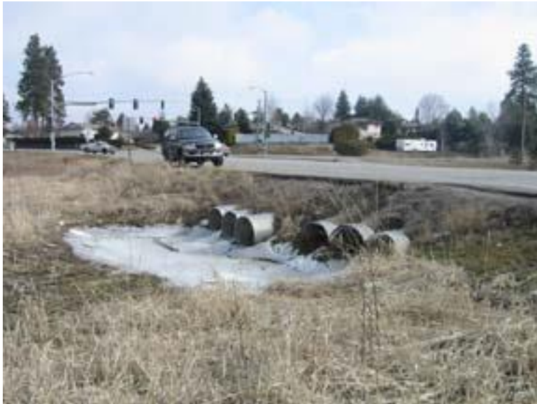
Figure 12: Dishman-Mica Road/Schafer Road. Looking at downstream face of culverts
