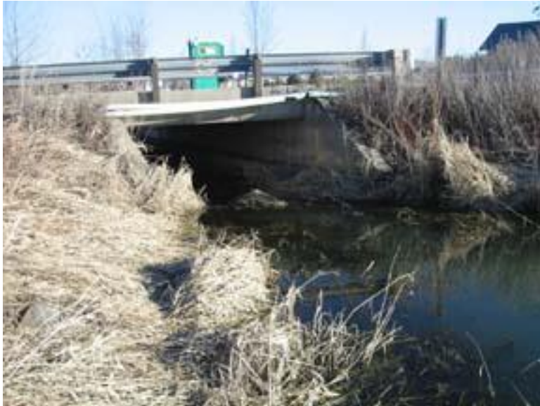
Figure 38: Thorpe road clear span. Looking at upstream bridge face
