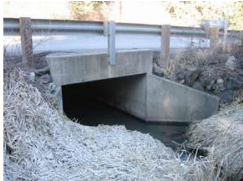
Figure 53: Dishman/Mica Road. Looking at upstream bridge face
