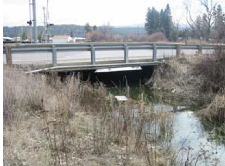
Figure 22: Bridge along Bowdish Road. Looking at downstream face
