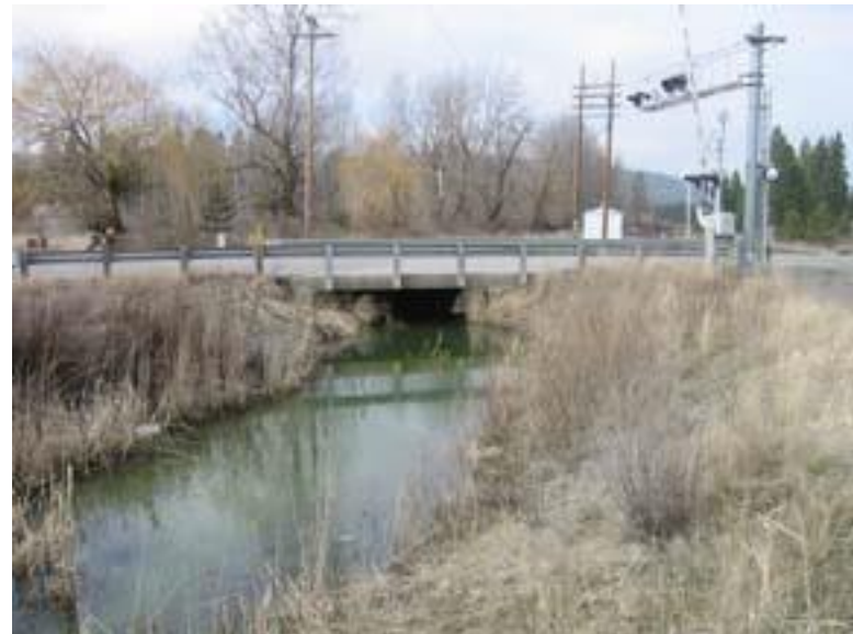
Figure 23: Bridge along Bowdish Road. Looking at upstream face
