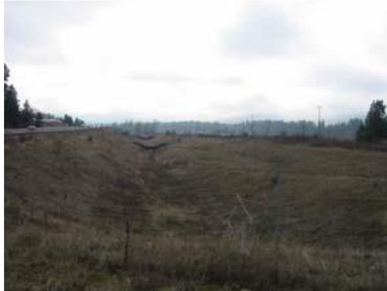
Figure 7: Dishman-Mica Road/28th Ave. Intersection. Looking upstream from 24th Ave.
