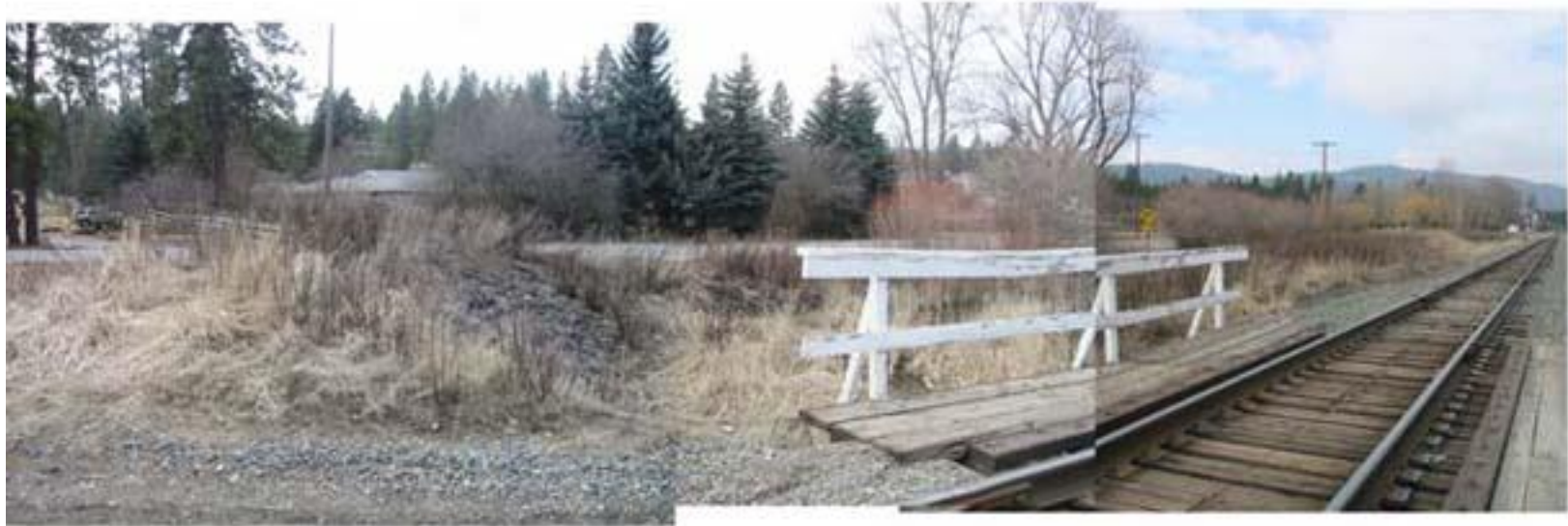
Figure 25: UPRR Bridge about 1/8 mile upstream of Bowdish road. Looking downstream
