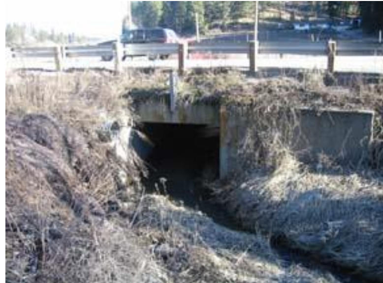
Figure 49: Dishman/Mica Road. Looking at upstream bridge face
