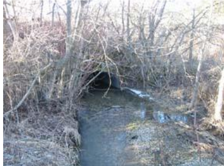
Figure 44: Mohawk road. Looking at downstream face of culvert
