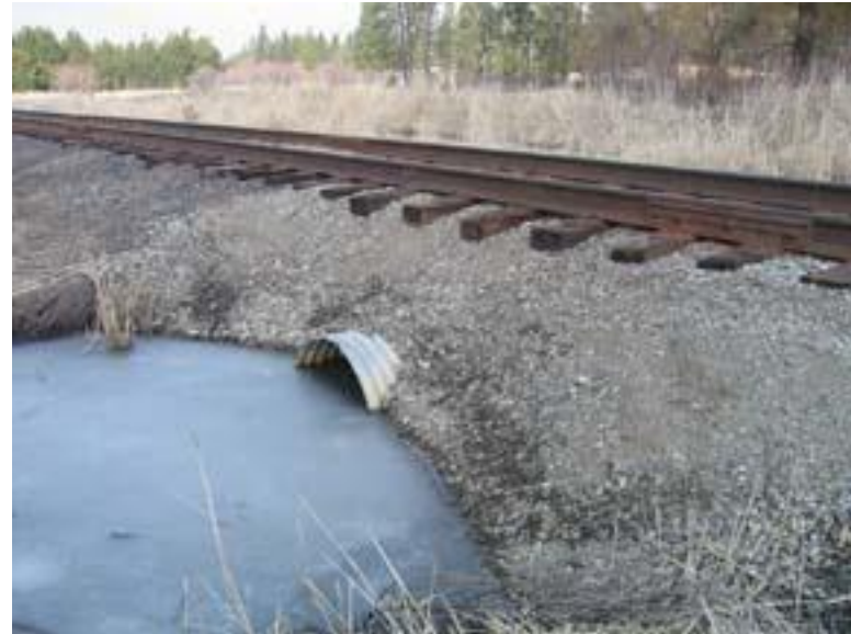
Figure 18: Culvert under railroad between Schafer and Dishman/Mica
