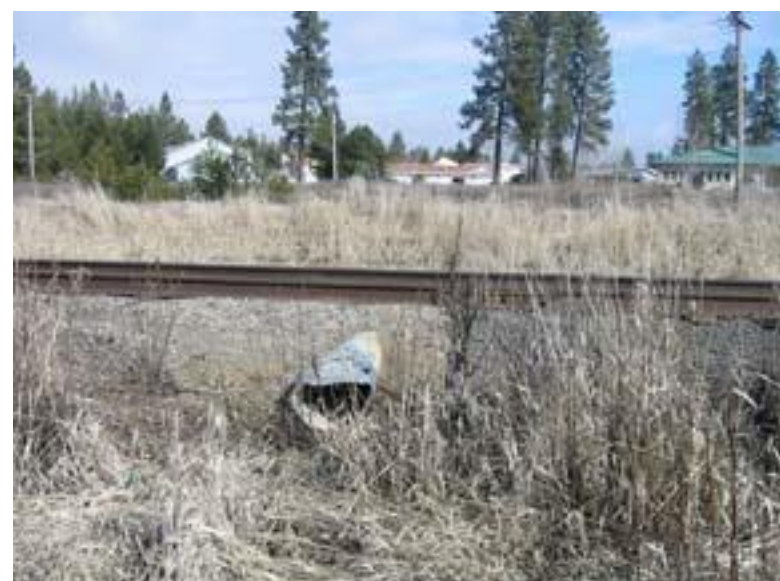
Figure 15: Culvert under railroad between Schafer and Dishman/Mica
