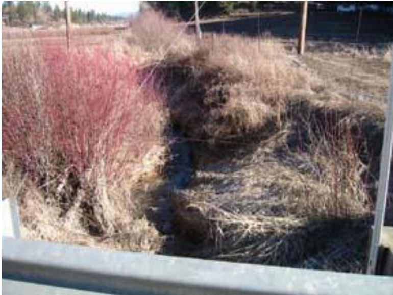
Figure 50: Dishman/Mica Road. Looking downstream
