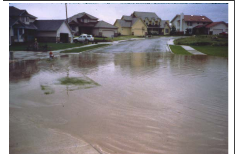
Figure 8. Post Construction Stormwater Drainage Problem
