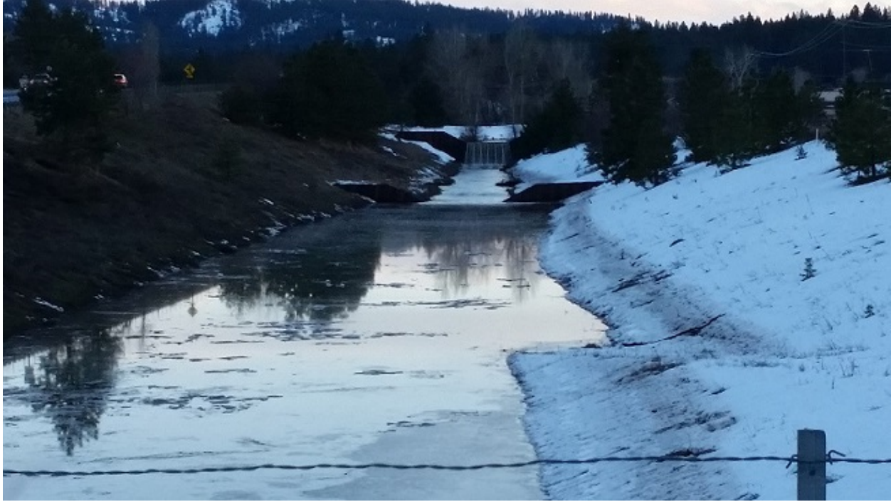
Incoming stream flow into retention ponds below Painted Hills project area during flooding
