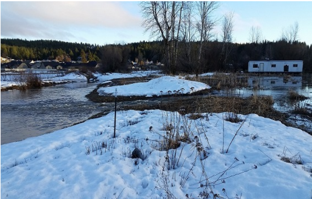
Incoming stream flow into Painted Hills project area during flooding
