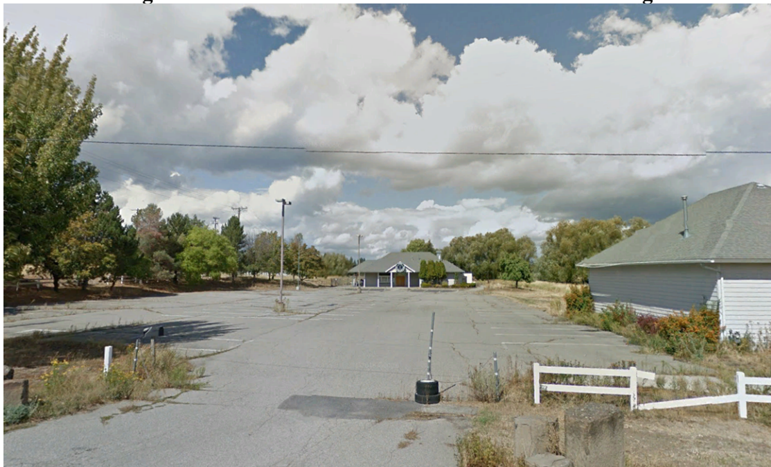
Figure 3-13: Former Clubhouse and Associated Parking
