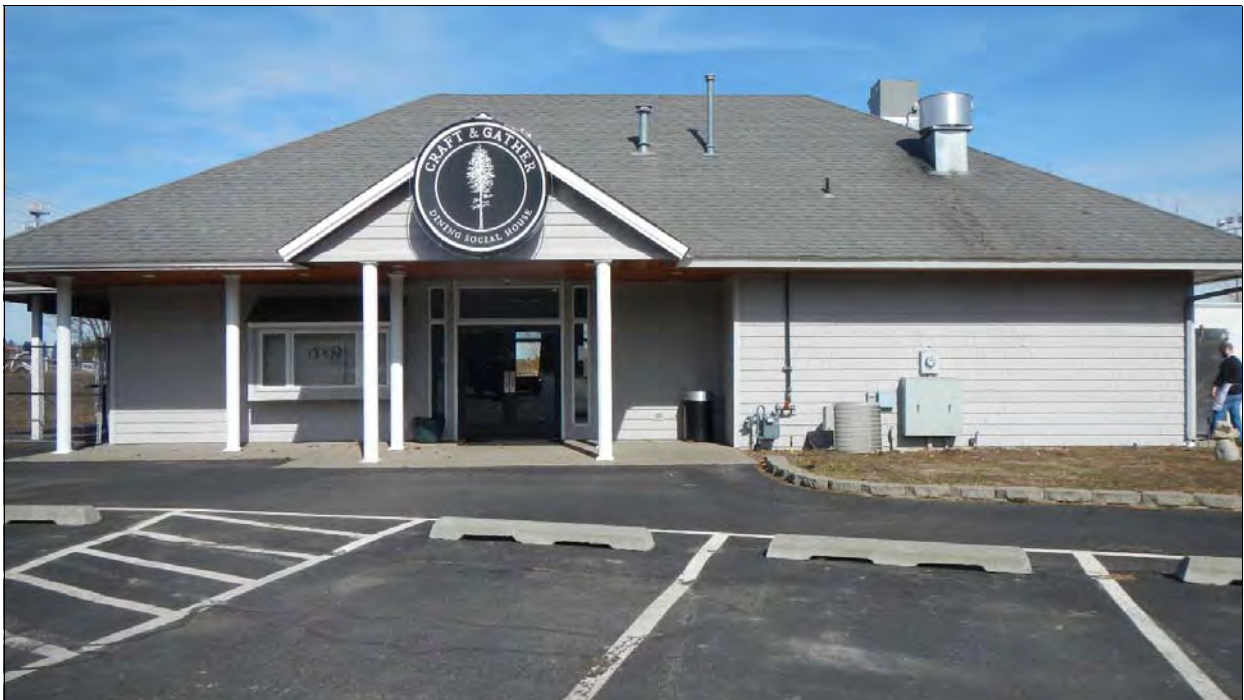
Figure 5. The Craft & Gather Café located in the southwest portion of the Project Area. View to the north.
