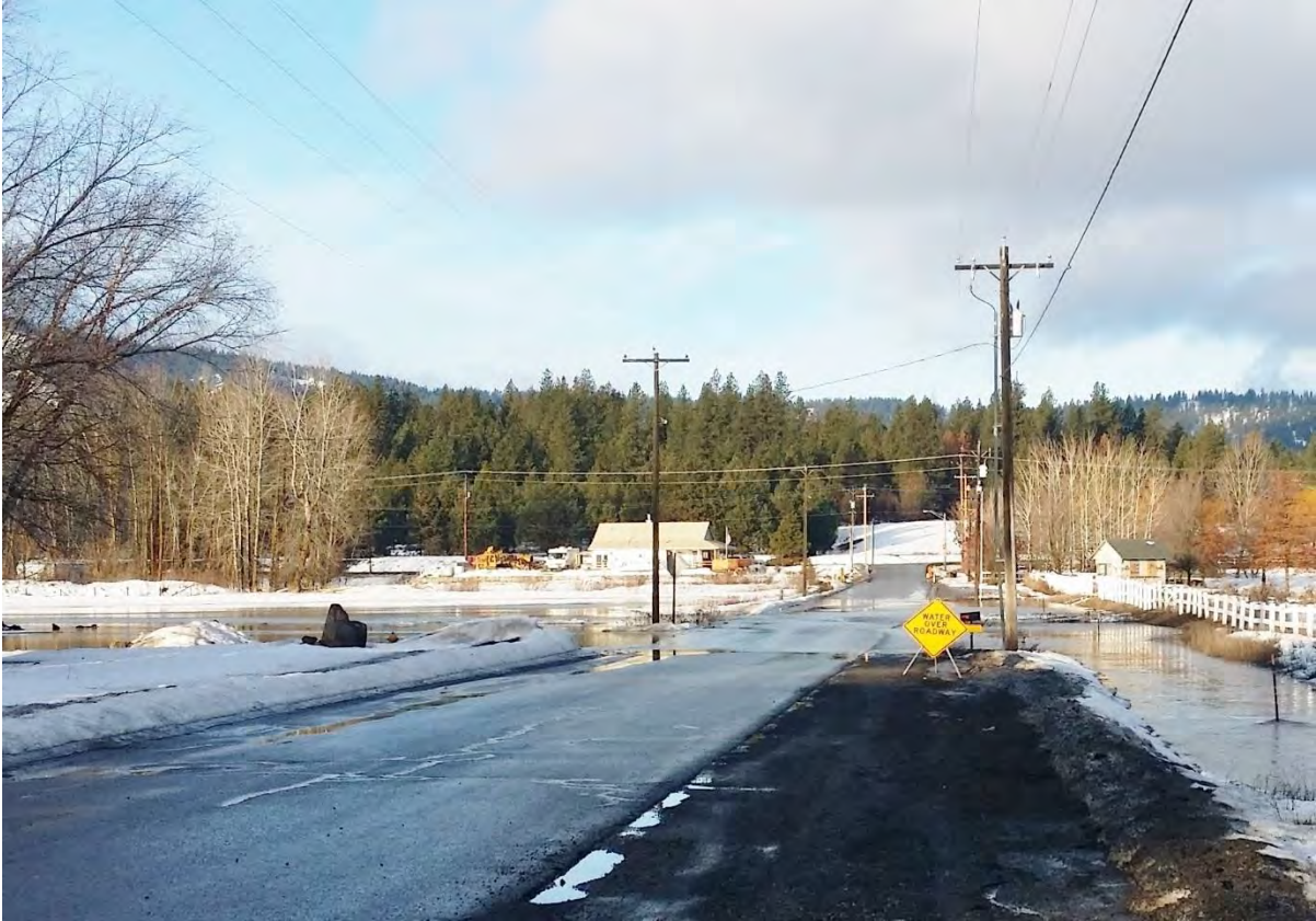
Figure 3-3: Flooding East of Chester Main Channel (Viewing Westward on Thorpe) 3
