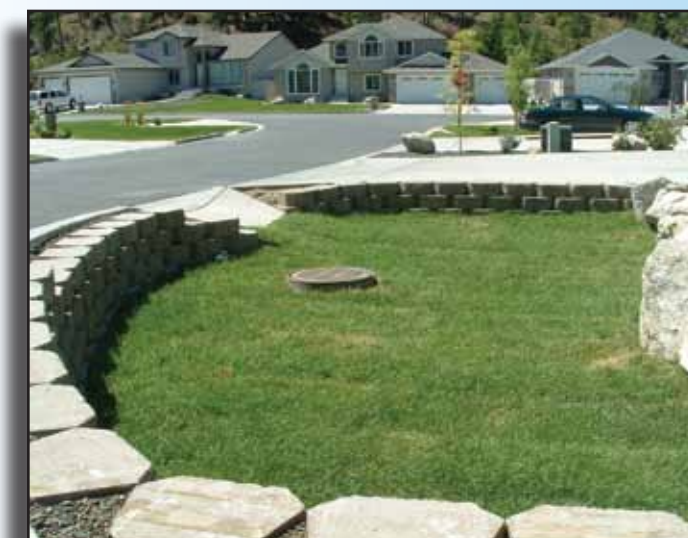
Stormwater swales and drywells recharge the Aquifer.
