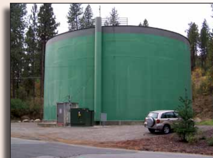
Public water purveyors pump & store Aquifer water.
