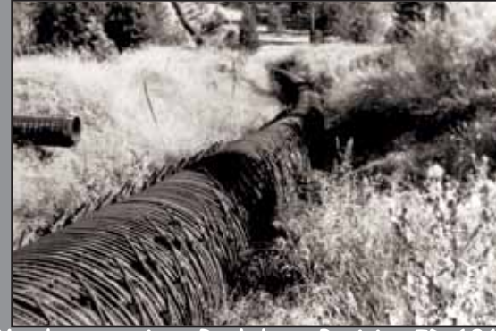
Wood stave pipe, Rathdrum Prairie, ID 1961
