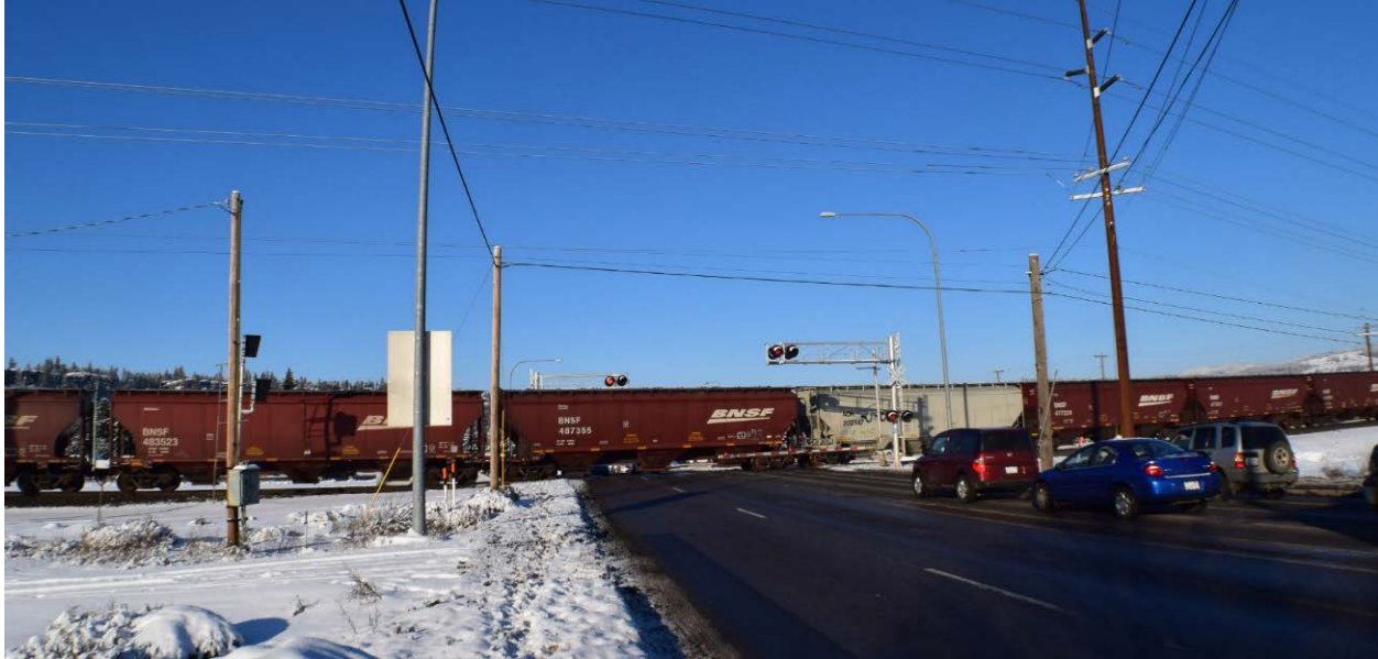
Figure 2: View of Existing Pines Road/BNSF Crossing
