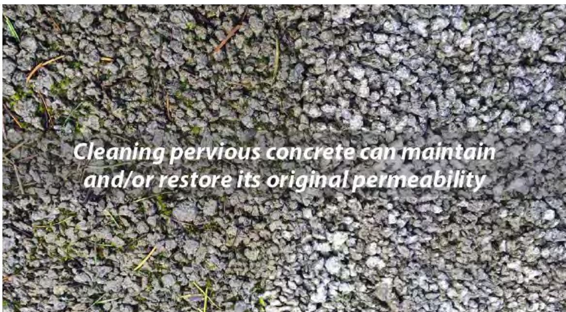
Figure 3: Comparison of PC that has and had not been maintained (NRMCA 2015).
