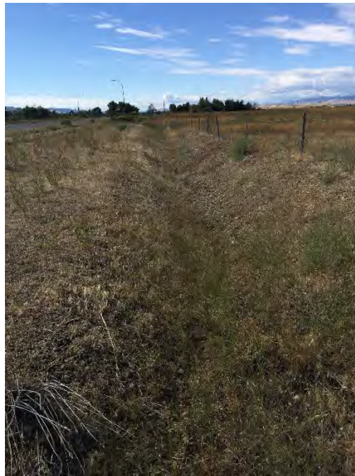
Figure 3.3 Biofiltration swale in EWA during the dry season
