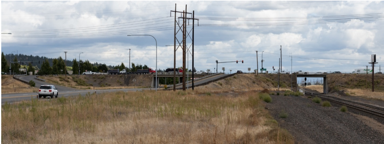
Figure 3: Sullivan Road Bridges Over Trent Avenue & BNSF Tracks
