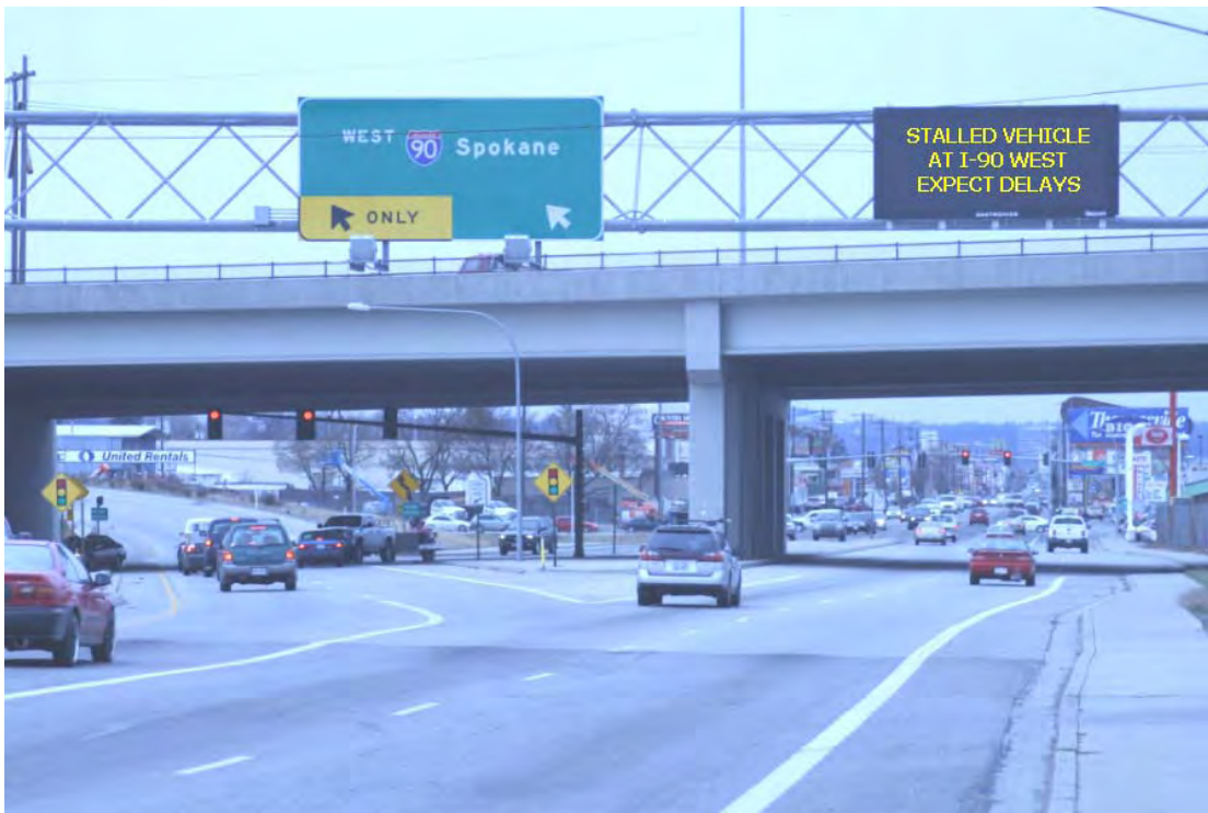
Front Access Dynamic Message Sign
